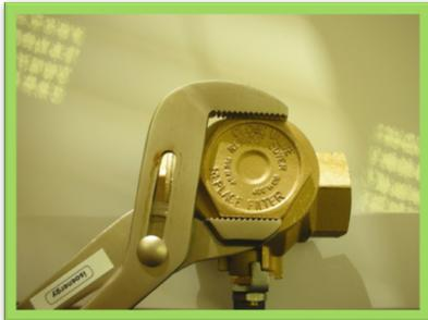
04. Remove filter inspection plug.
