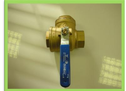
03. Adjust large pliers to maximum size and unscrew the filter inspection plug on top of the valve.
