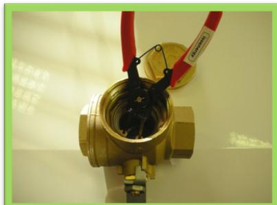
08. Replace plug and tighten with large pliers before finally moving the handle back to the "ON" position.
